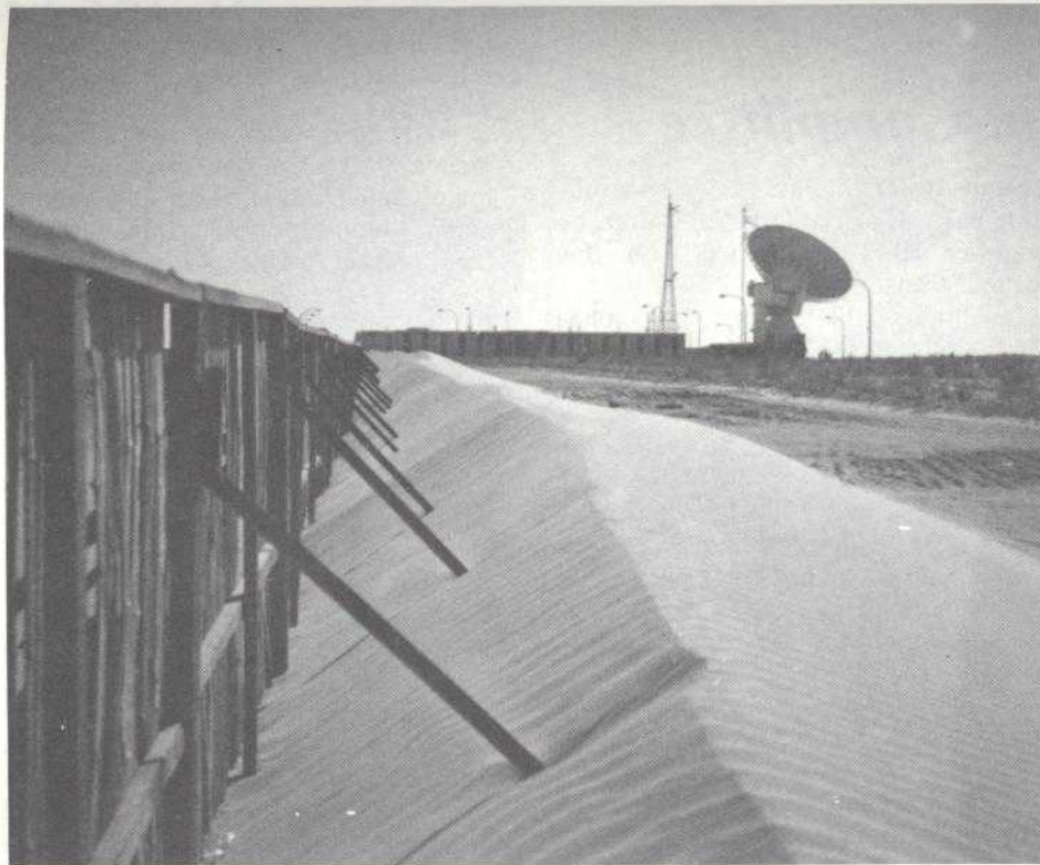
Sand barriers at Umm Al-Aish.
