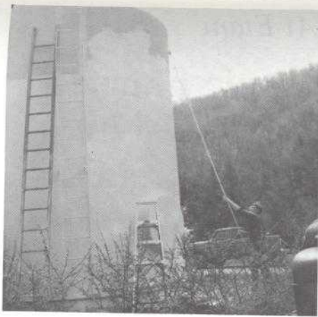
Andy Thomson paints Etam Water tank with a long-handled roller.
