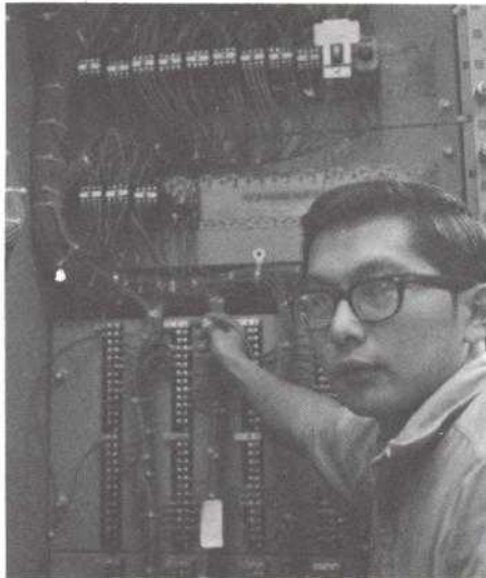
Mechanic Harvey Fujimoto repairs the emergency start switchgear.
